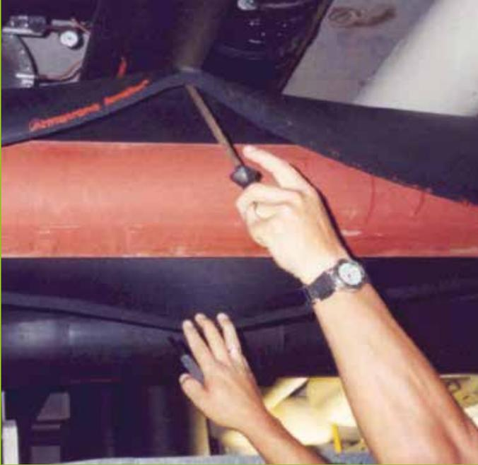
*Fig 7: This cold water pipeline has been protected by Armaflex for 20 years - the picture shows maintenance inspection of the original system.*
