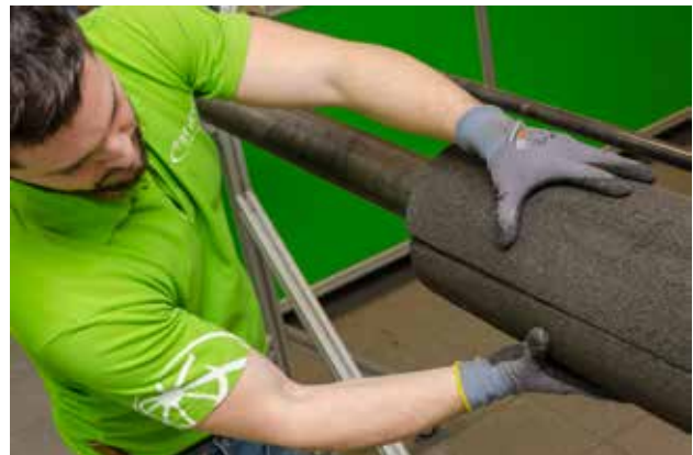
Cellular glass is installed with a two-component adhesive and then additionally secured with installation tape or metal straps.
