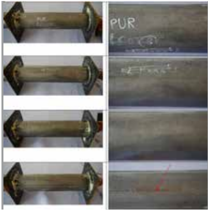
Figure 14: Pipe surface of Sample D, polyurethane, after 65 days.
