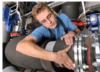
Installing acoustic solutions.
