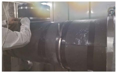
Figure 13: Installation of the Acoustic Barrier
