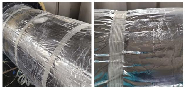
Figure 10: Repair of superficial damage. Left: spray adhesive, right: aluminium adhesive tape
