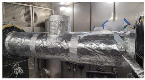
Figure 11: Installation of the vapour barrier
