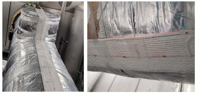
Figure 12: Sensor for humidity detection. Left: sensor at 12 o'clock, right: sensor at 6 o'clock
